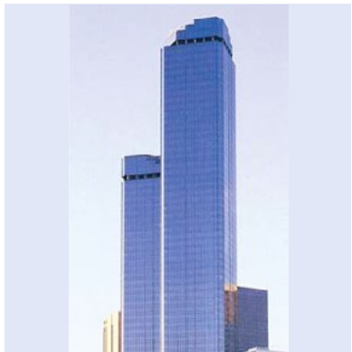
“Administration building”, Melbourne, Australia
